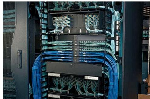
**Figure 6. PANDUIT® QUICKNET™ Angled Modular Patch Panels and Cabling Assemblies reduce deployment times and optimize space in dense patching environments.**
